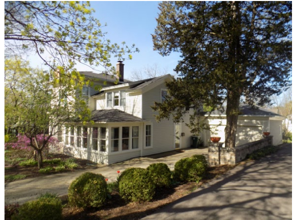
2016 – 501 South Street and Garage
