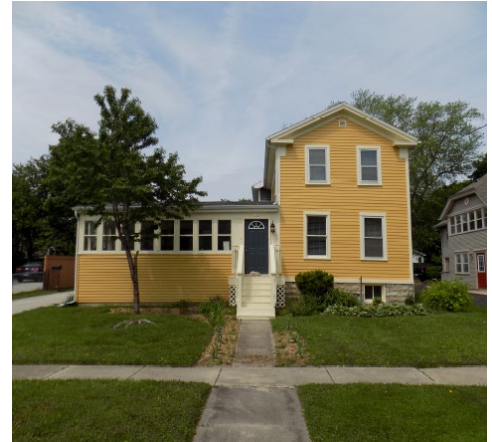
2016 – front façade / Fifth Street
