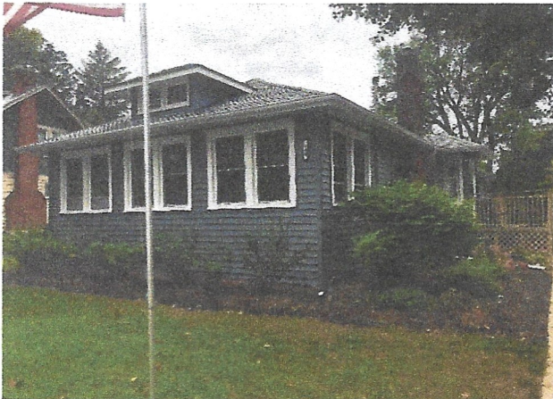
Figure 1 Front of 140 N Harrison St
