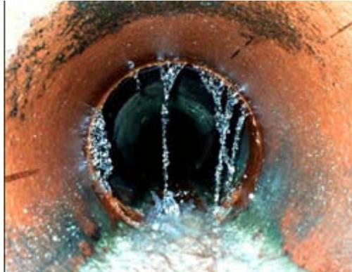
*Above is an example of storm water entering into the sewer system from a manhole (left) and from a defect inside a pipe (right).*
