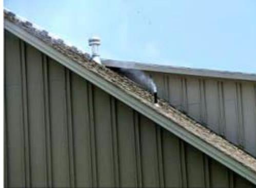
Roof vents are where the smoke should be released or seen. This is good!
