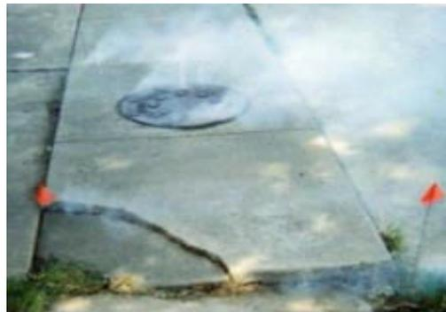
*High-capacity blowers are used to pump smoke into a manhole (left photo). In the right photo, smoke is pushed into the system and emerges from cracks in the sidewalk and at a downstream manhole.*
